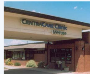
Photos courtesy CentraCare
